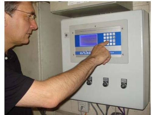
The projected effect of installing a master control was calculated by using a simulation program. In this example, the simulation program projected energy savings of 29.1% based on eliminating unload time energy and lowering the system pressure. After the installation of the master control it was necessary to evaluate the actual results for the system over a period of one week.
